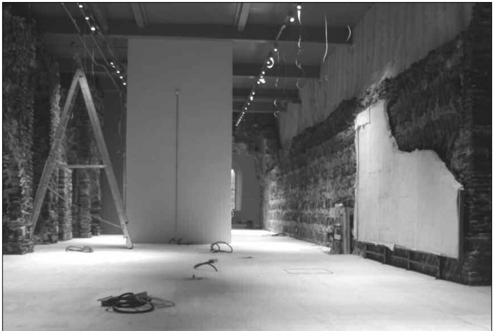
East Gallery, building works completed, 14th November
